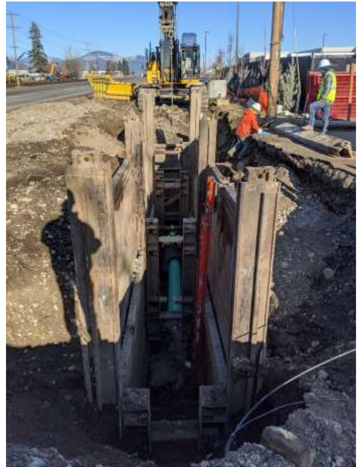
Hwy41 Upsizing Water & Sewer Lines
