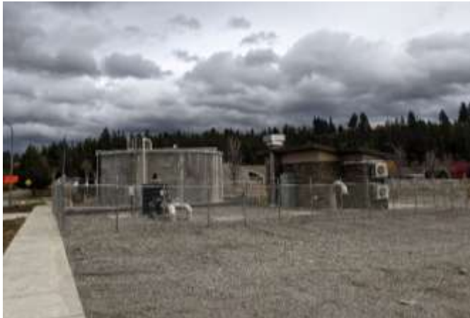
12 th Ave EQ & Lift Station
