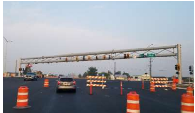
Hwy41 Traffic Signals
