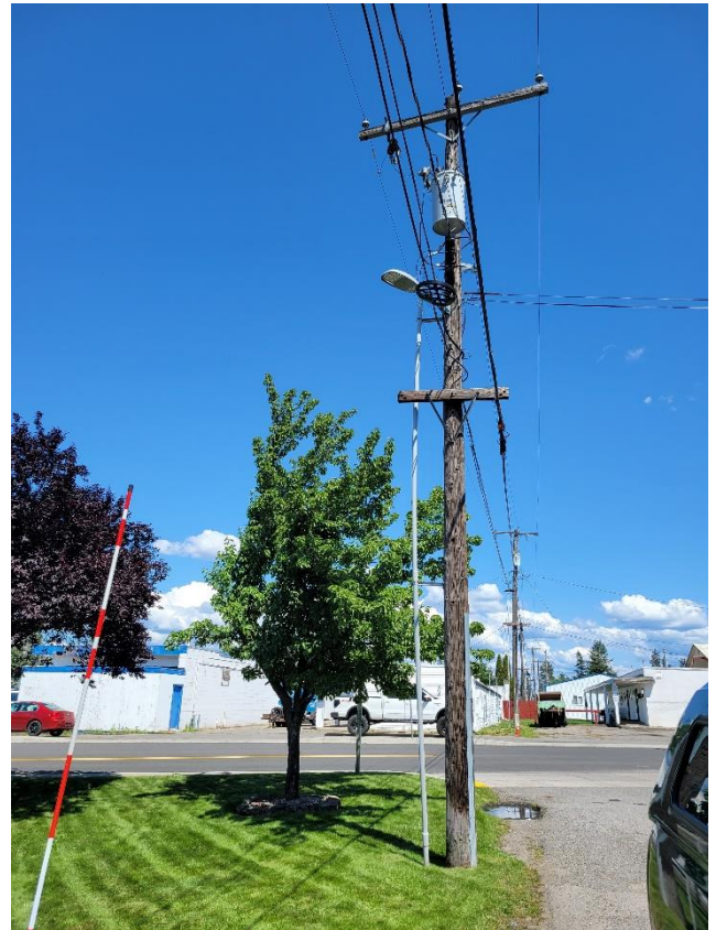
Powerline (Avista) - looking eastward to project site (2)
