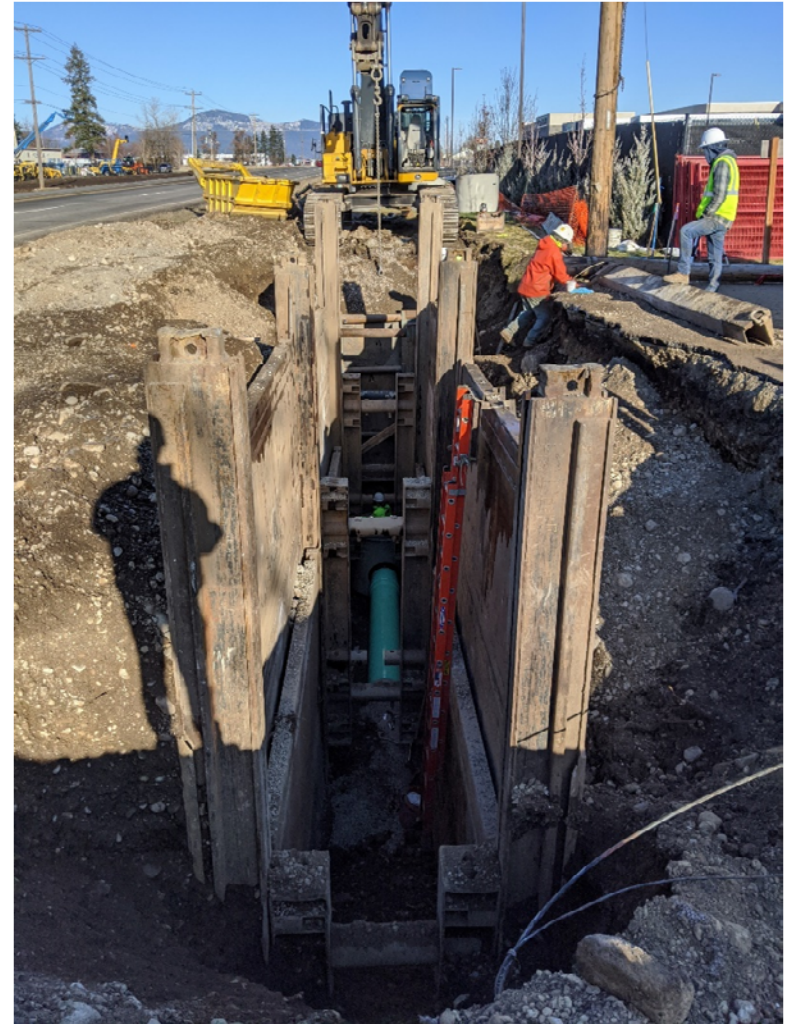
Hwy41 Upsizing Water & Sewer Lines
